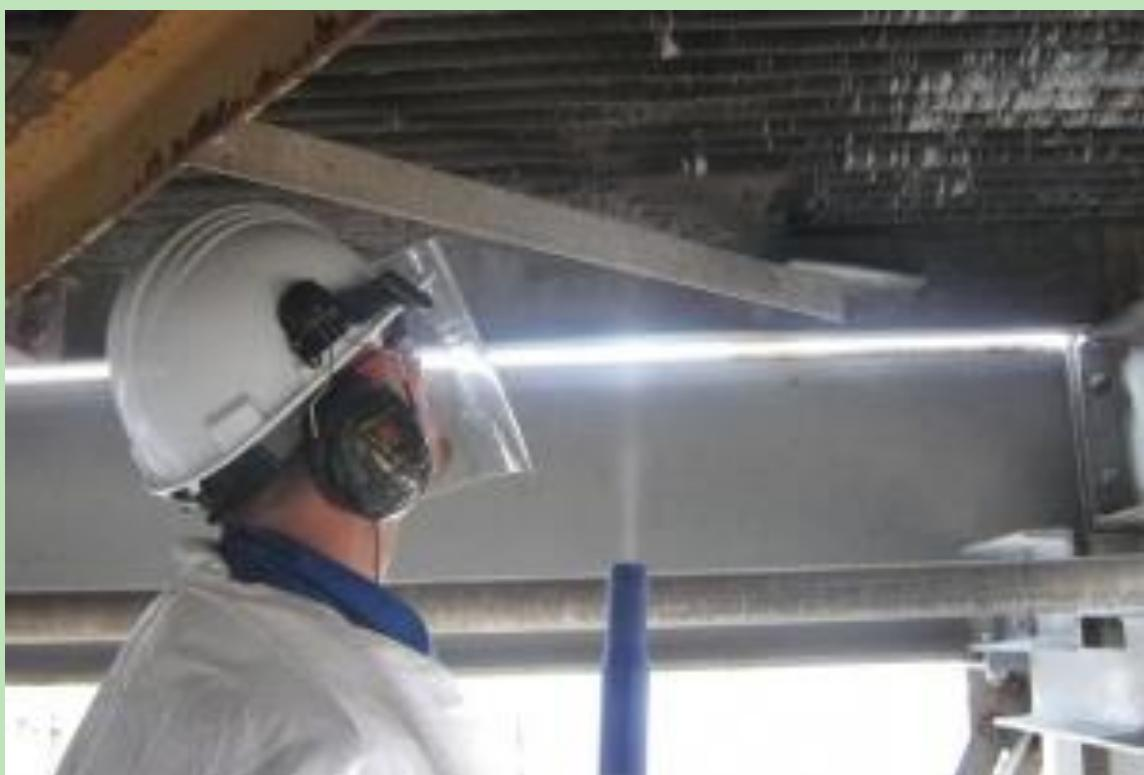
Dry blasting with sodium bicarbonate is a very soft blasting method which does not heat or wet the surface.
